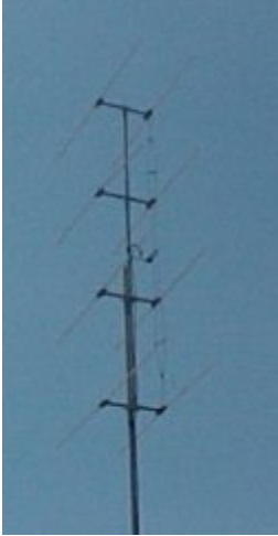
Figure 8. - Four stacked half wave dipoles collinear antenna
